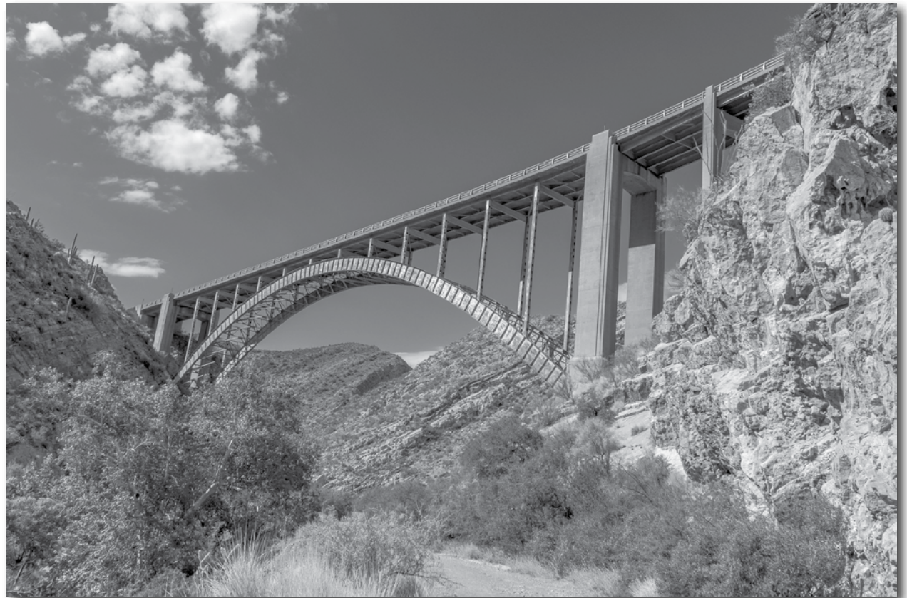
Construction begins soon on Queen Creek Bridge replacement.
